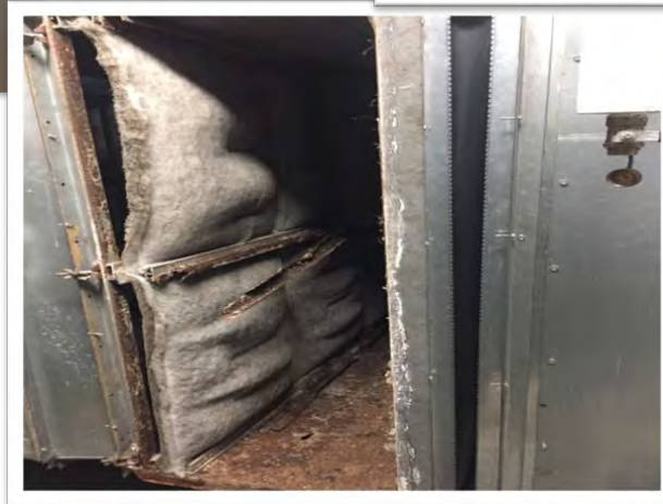
Mechanical systems (installed 1992) have exceeded standard life span of 20 to 25 years.
