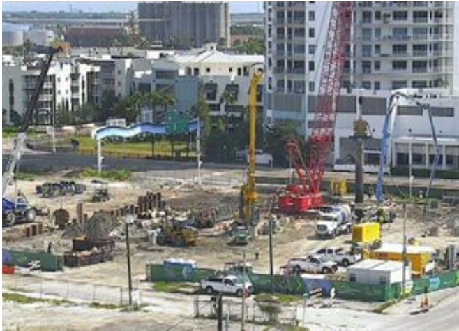
September 27, 2017 Installation of deep foundations (caissons)
